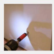
**5.** While holding the boards in position drill 9 80mm depth holes through the SoundBoard 4 into the wall behind.
