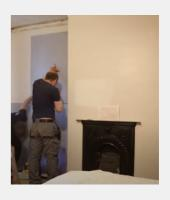
**4.** Offer your first board to the wall making sure it sits square **leaving a 5mm gap around the perimeter edge of the wall, floor and ceiling.** You may need to scribe the boards to follow the curvature of your surrounding walls, floor and ceiling to maintain the 5mm gap.
